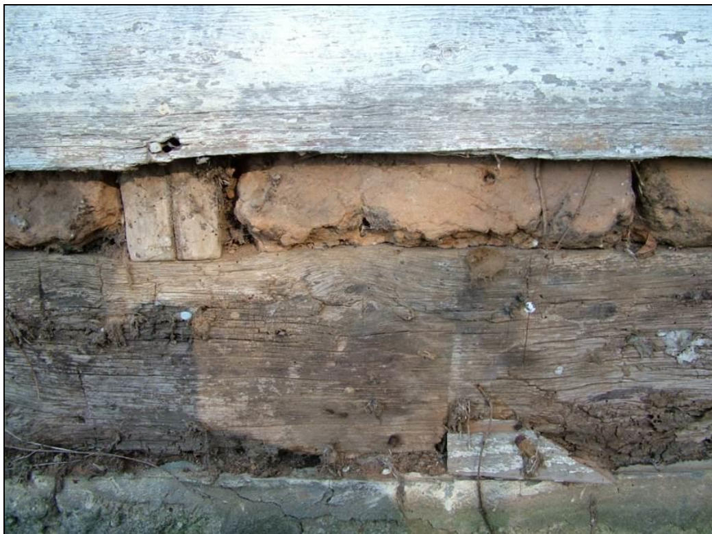
Photo 30: Clay Nogging on Sill and Siding of the Duplex.
