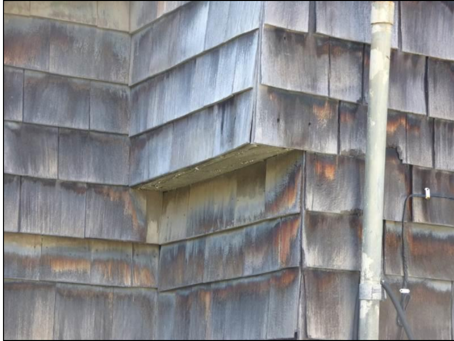
Photo 45: Jettied Construction Detail on Northeast Elevation.
