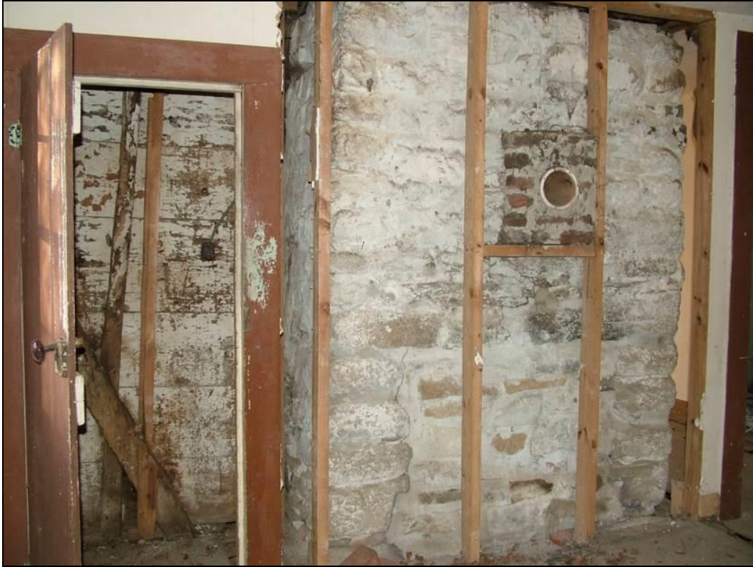
Photo 31: Infilled Fireplace and Stove Hole in the Duplex.
