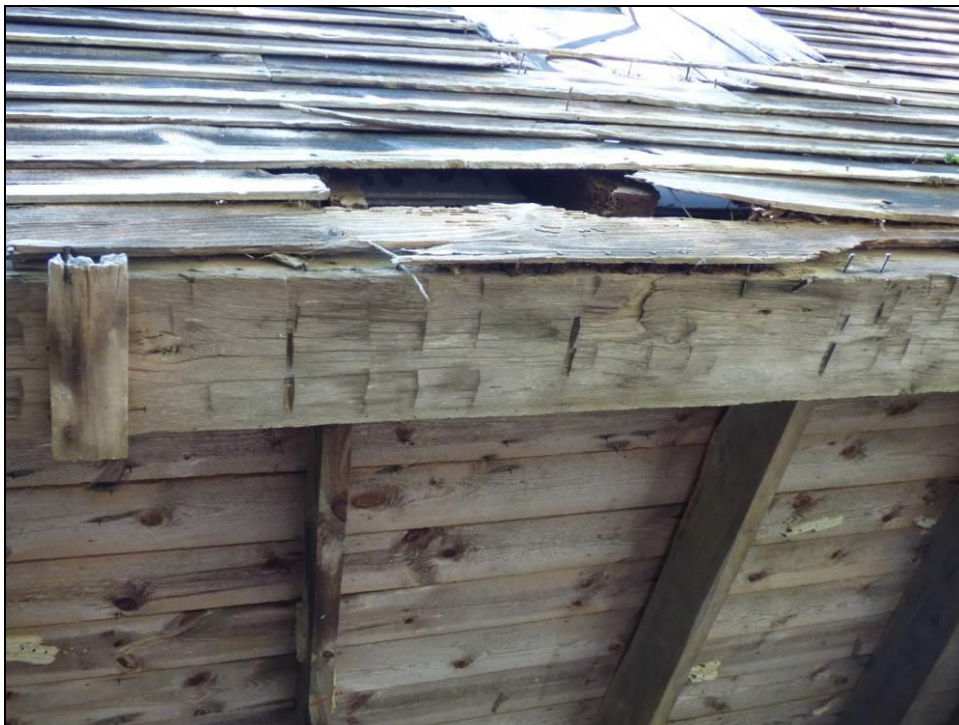
Photo 110: Saw and Adze Marks on Southwest Elevation.
