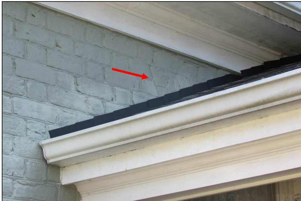
Photo 60: Splayed Jack Arch on Southwest Elevation Noting an Original Fenestration.
