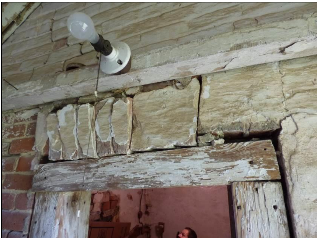
Photo 77: Spring House, Jack Arch Detail on Interior.
