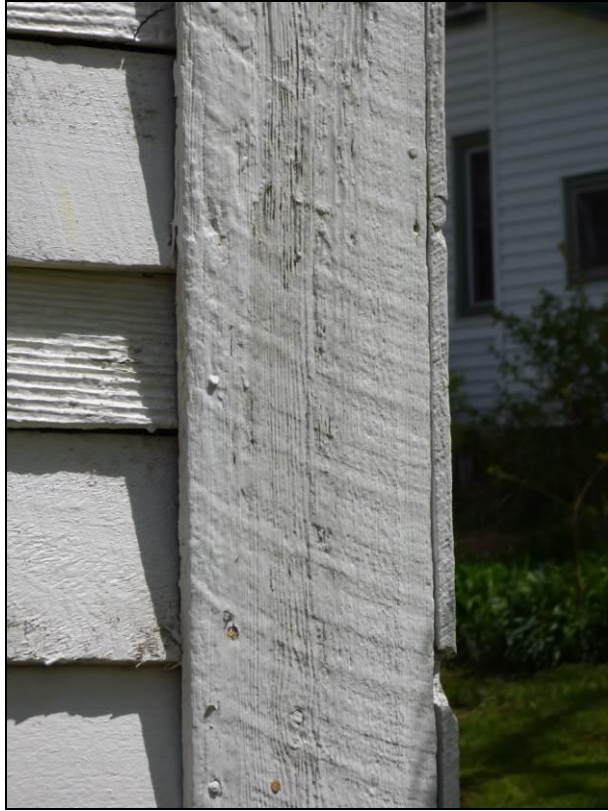
Photo 82: Circular Saw Mark Details on Northeast Elevation.
