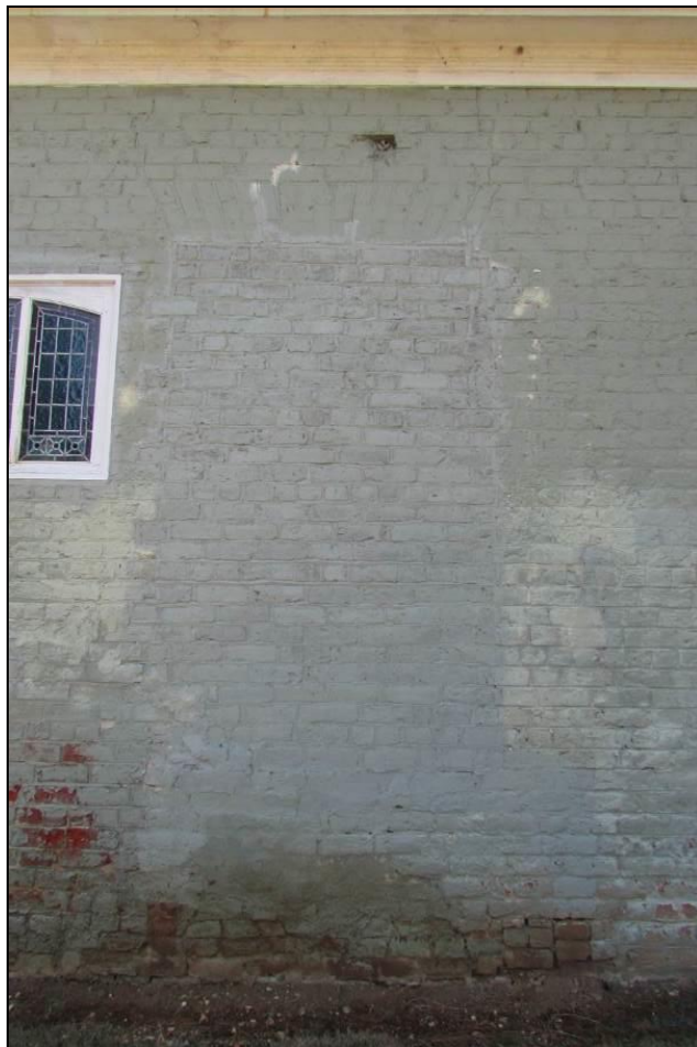
Photo 58: Splayed Jack Arch and Brick Scarring on Northeast Elevation Showing an Original Entry Location.
