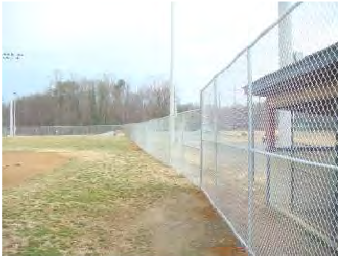
New sideline fence and outfield fence
