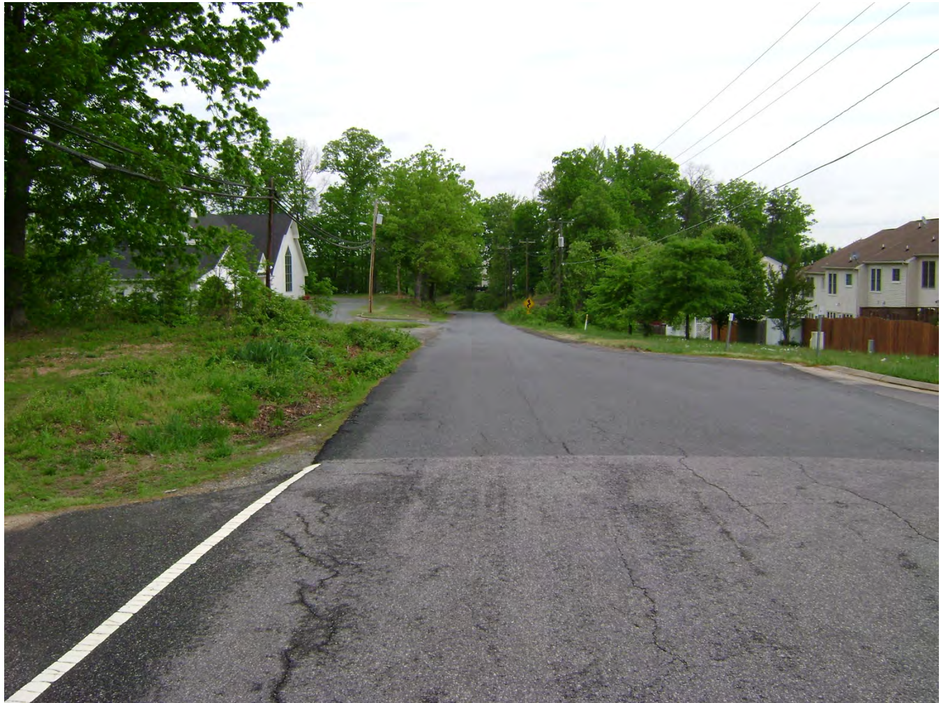
Bells Hill Road – Phase 1
