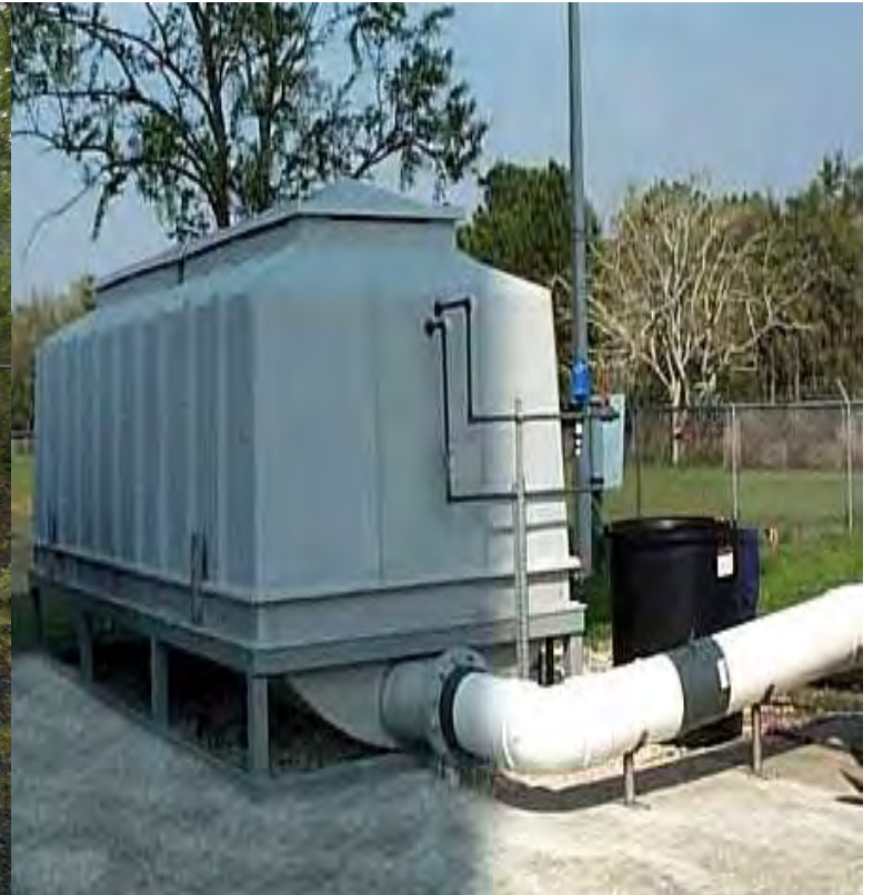
Falls Run SPS - Typical Biofilter Unit by Envirogen Technologies
