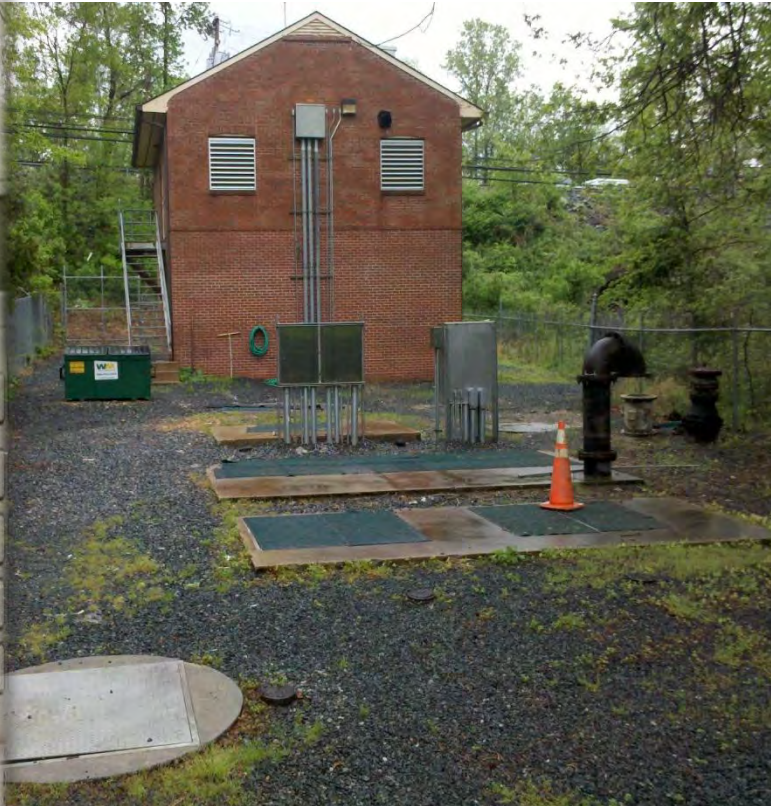
Falls Run SPS - Typical Biofilter Unit by Envirogen Technologies
