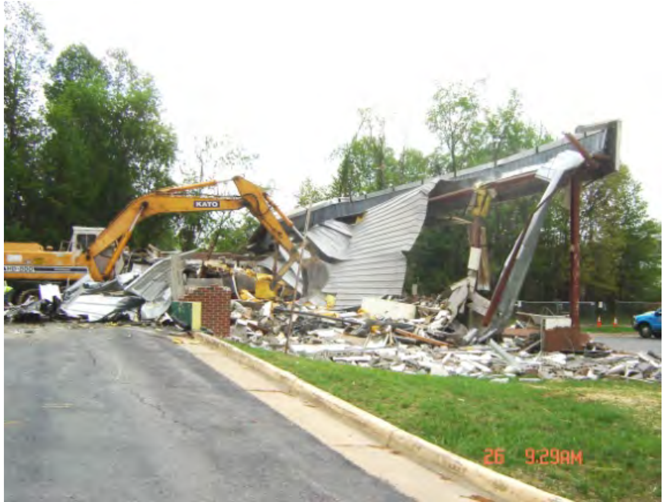
Demolition of Rescue 1 Building
