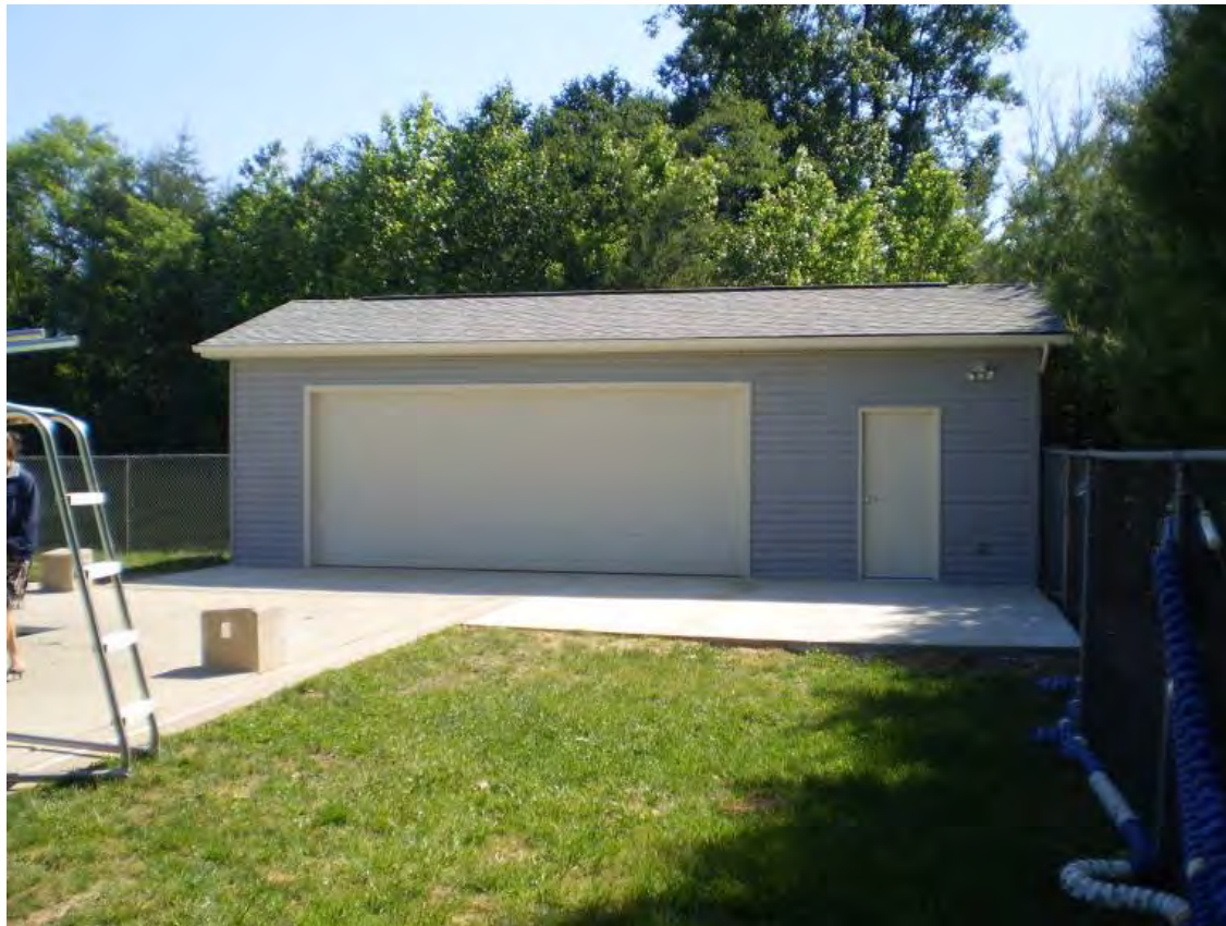
New storage building
