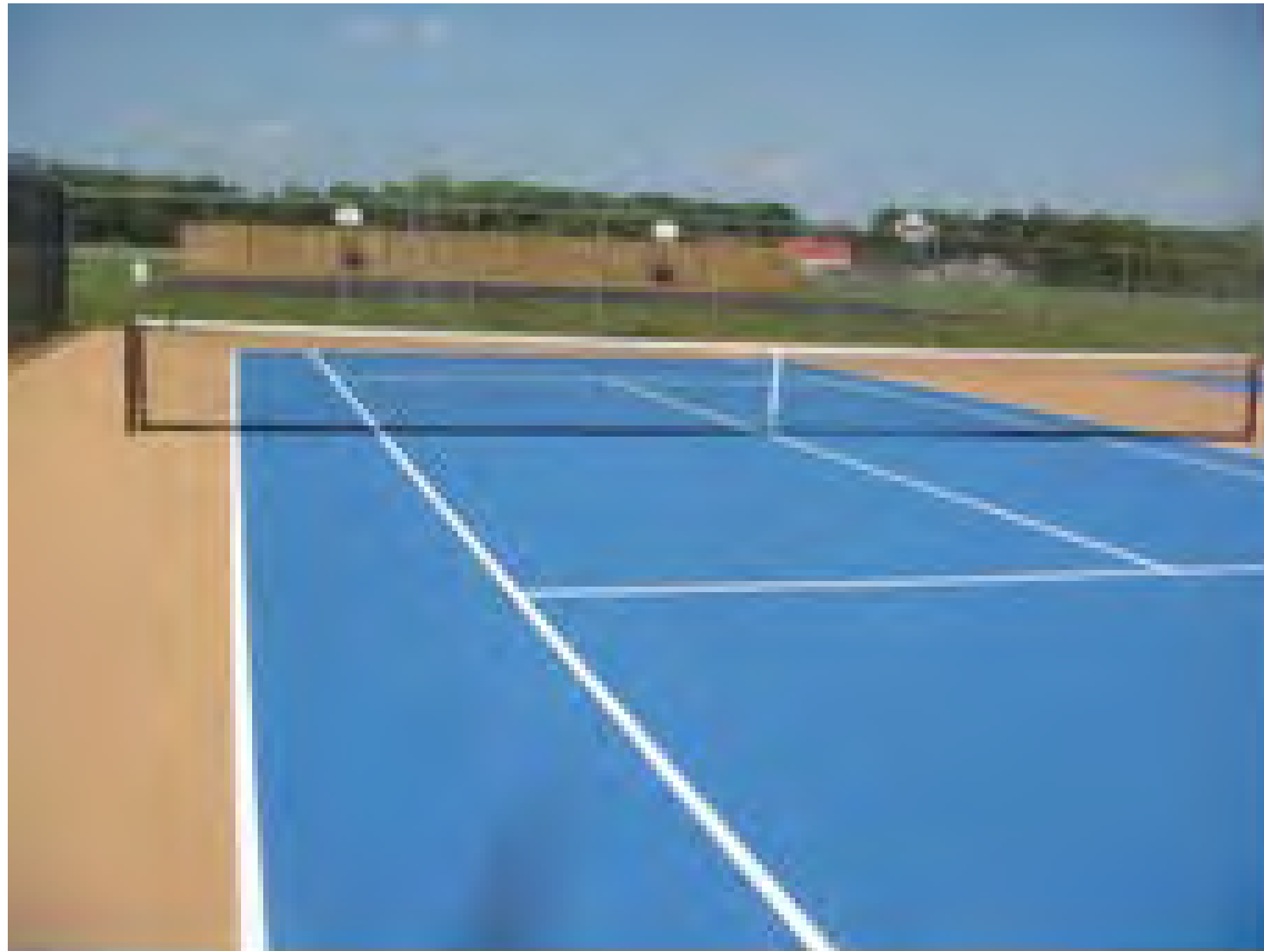
Tennis courts after repairs
