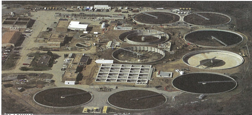
Upgrades to the Aquia Wastewater Treatment Facility continued throughout 2010 to meet more stringent nutrient removal requirements and expand the facility's treatment capacity to 10 million gallons per day.
