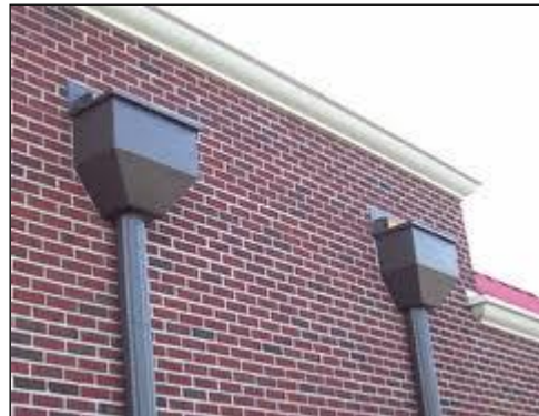
Scuppers collect rainwater from flat roofs behind parapet walls
