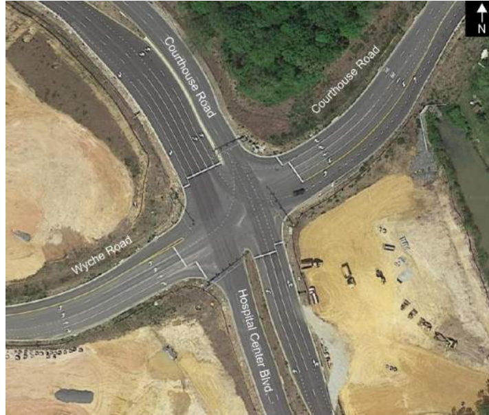
Figure 7. Aerial of Courthouse Road/Hospital Center Blvd. and Wyche Road/Courthouse Road
