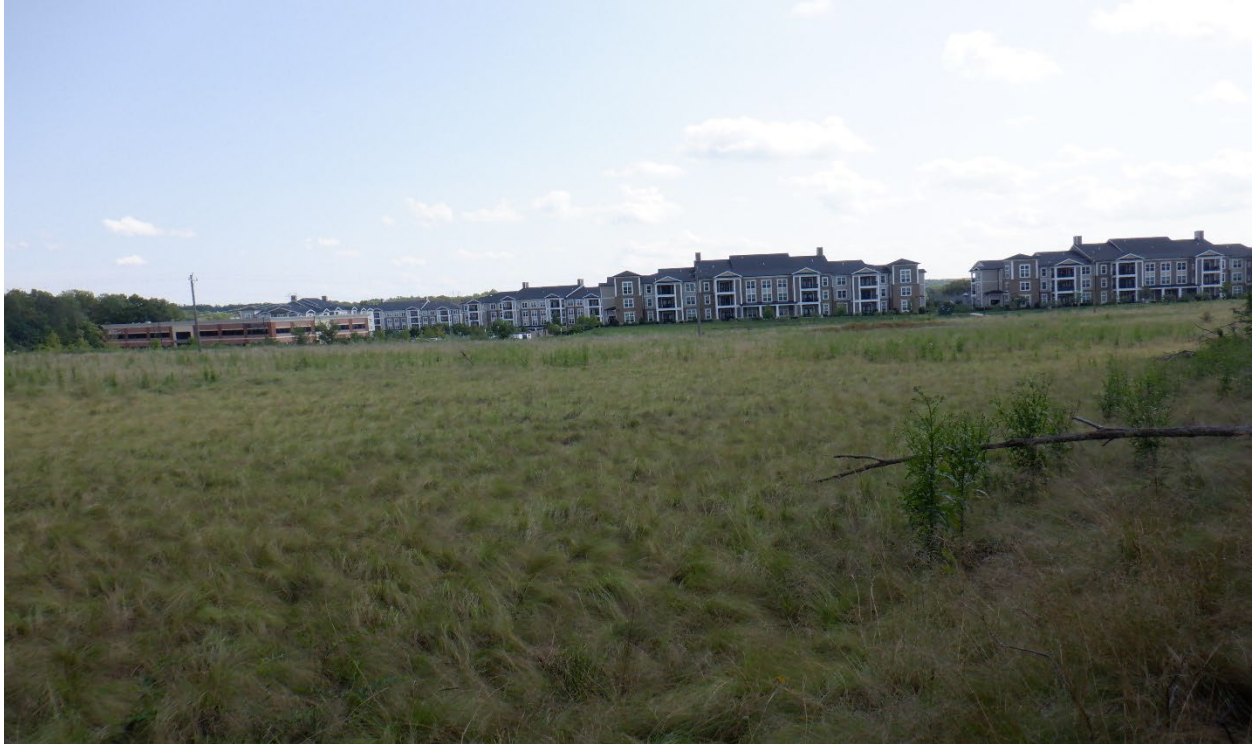
Photograph 5: The Site consists of recently cleared and graded areas.
