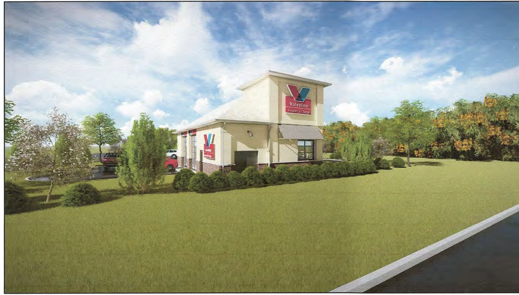
VIEW FROM GARRISONVILLE ROAD LOOKING TOWARDS THE EAST/NORTHEAST
