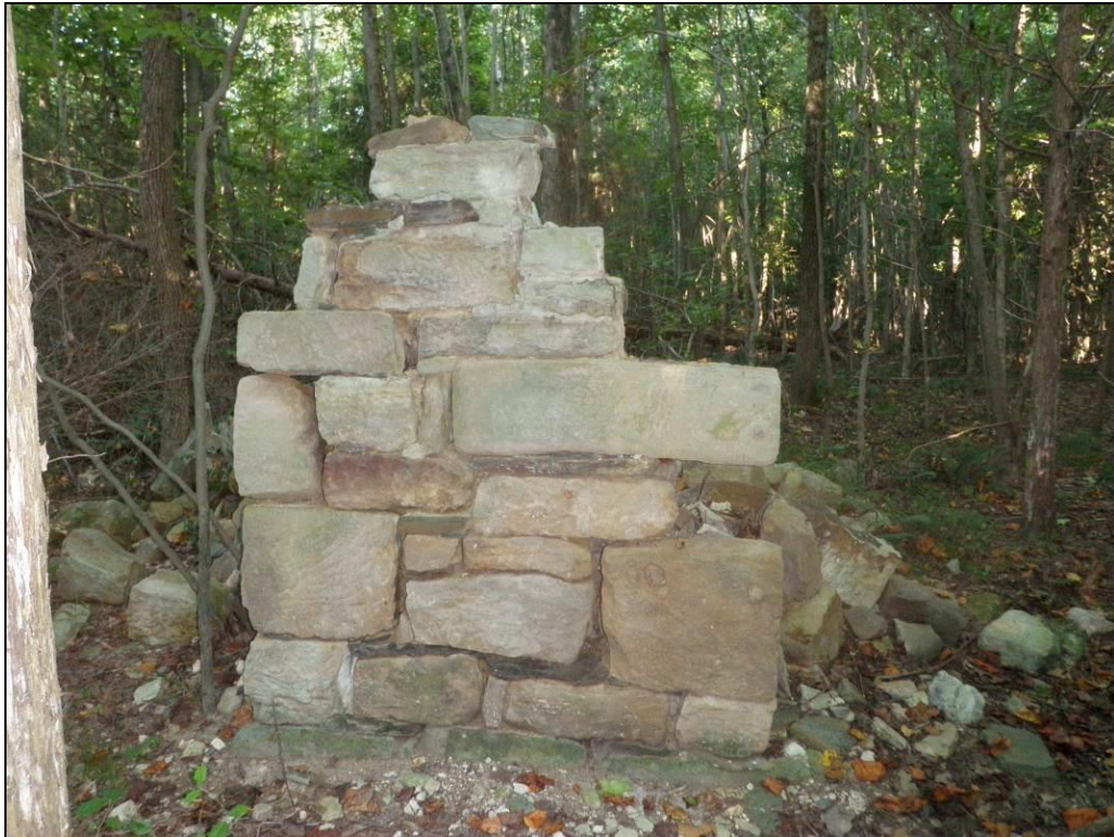
Photo 7: View West Showing the Construction of the Chimney on Site 44ST1221.
