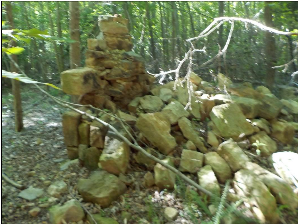
Photo 6: View East Showing the Chimney Remains.
