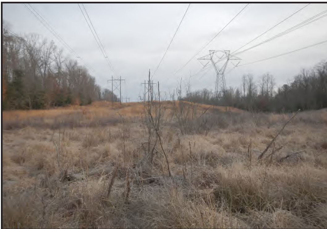
Figure 12. Photograph taken from ST N925 E1525 looking north, showing wet area with dry grasses in the foreground, hardwoods on either side of the powerline corridor; and powerlines in the background
