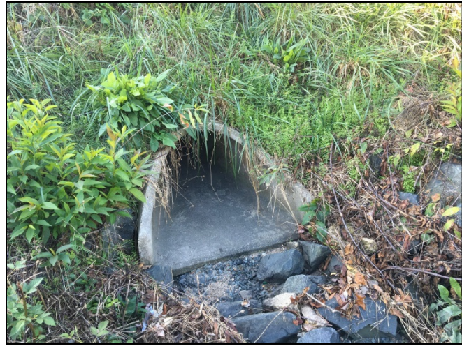
Figure 1. Stafford County MS4 Outfall Node ID: CO-RPR(1)1 located off Village Parkway
