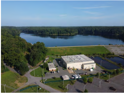
SLWTP-001 Smith Lake WTP Filter Repairs Phase 3
