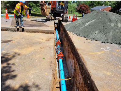
3R Water Distribution System Rehabilitation Small Water Projects
