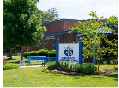
Hartwood Elementary Rebuild
