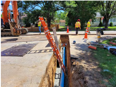
3R Water Distribution System Rehabilitation Neighborhood Systems
