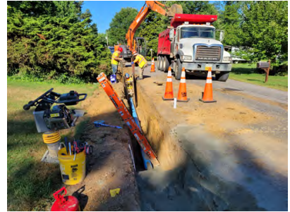
3R Water Distribution System Rehabilitation Transmission Lines
