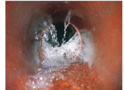
An offset pipe joint showing active Infiltration/Inflow was located during a TV inspection.
