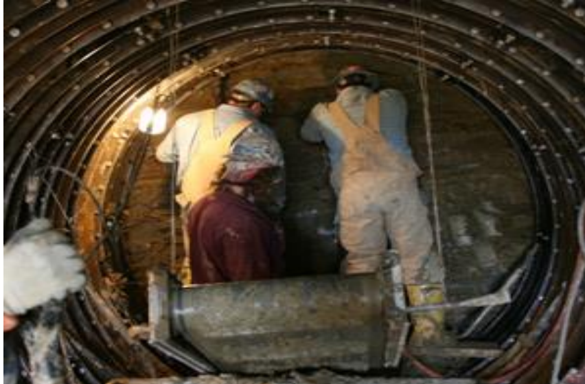
Example of setting shot for tunnel blast
