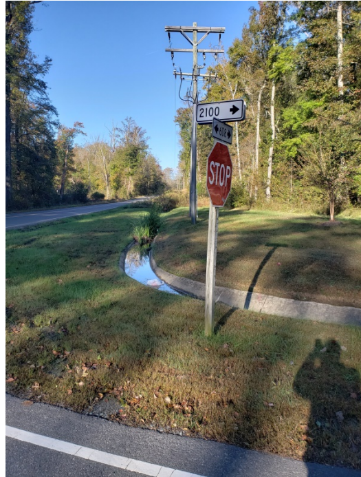
Brooke Road – Crestwood Lane Intersection Standing Water & Paved Swale-Ditch Maintenance Needs
