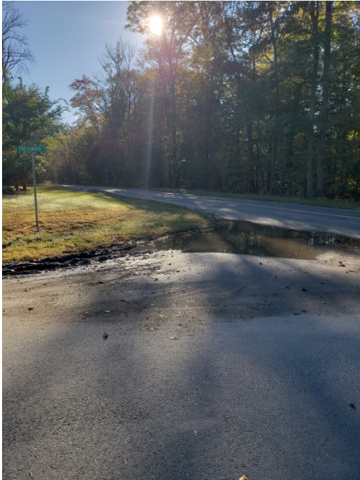
Brooke Road – Crestwood Lane Intersection Standing Water & Paved Swale-Ditch Maintenance Needs
