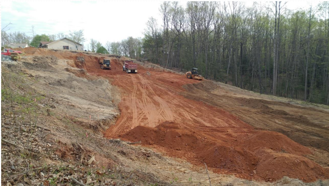
Mass grading and foundation preparation
