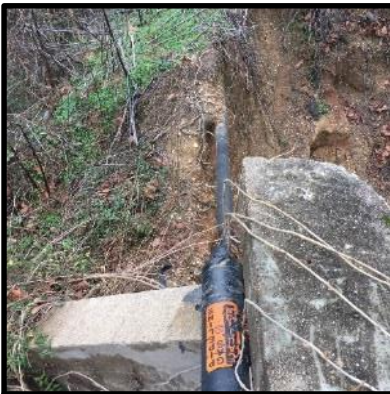
Exposed natural gas line at Old Dairy Lane Bridge abutment at Clairborne Run
