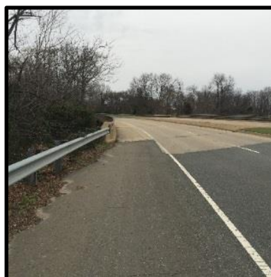
Facing north on Rt. 3 at the CSX RR overpass. The shoulder width is less than 8'.
